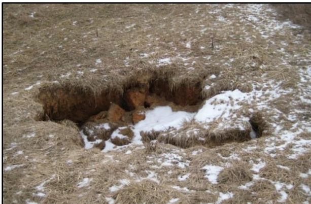
Figure 7-3: Sinkhole on Airport Property
